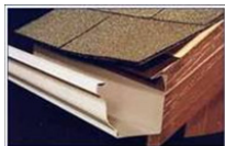
Tuck gutter under existing drip-edge
